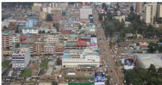
Figure 2: Aerial view of Langas Estate (Olengwe, 2018)
